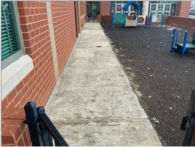
ACCESSIBLE ROUTE TO PLAYGROUND
