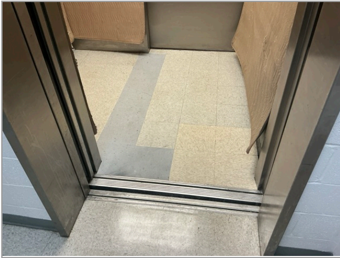
LOBBY LOOKING AT CABS (WITH DOORS OPEN)
