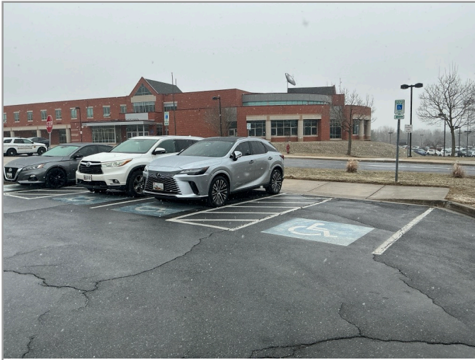
OVERVIEW OF ACCESSIBLE PARKING AREA
